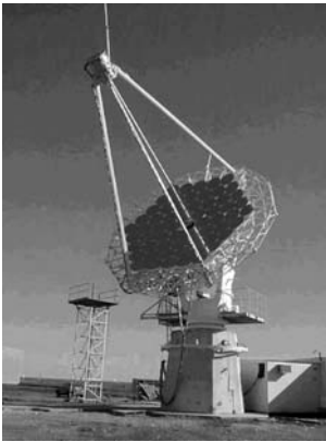
Fig. 6.43 Photograph of the air Cherenkov telescope CANGAROO (CANGAROO – Collaboration of Australia and Nippon (Japan) for a GAMMA-Ray Observatory in the Outback) [15]
